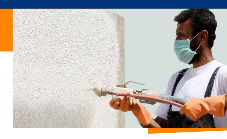
Ressichem Dry Mix mortars / Premix Plasters are factory manufactured dry mortars confirming to specific mix proportions of ingredients e.g., Binders, Aggregates, fillers, pigments, chemical additives, etc.
