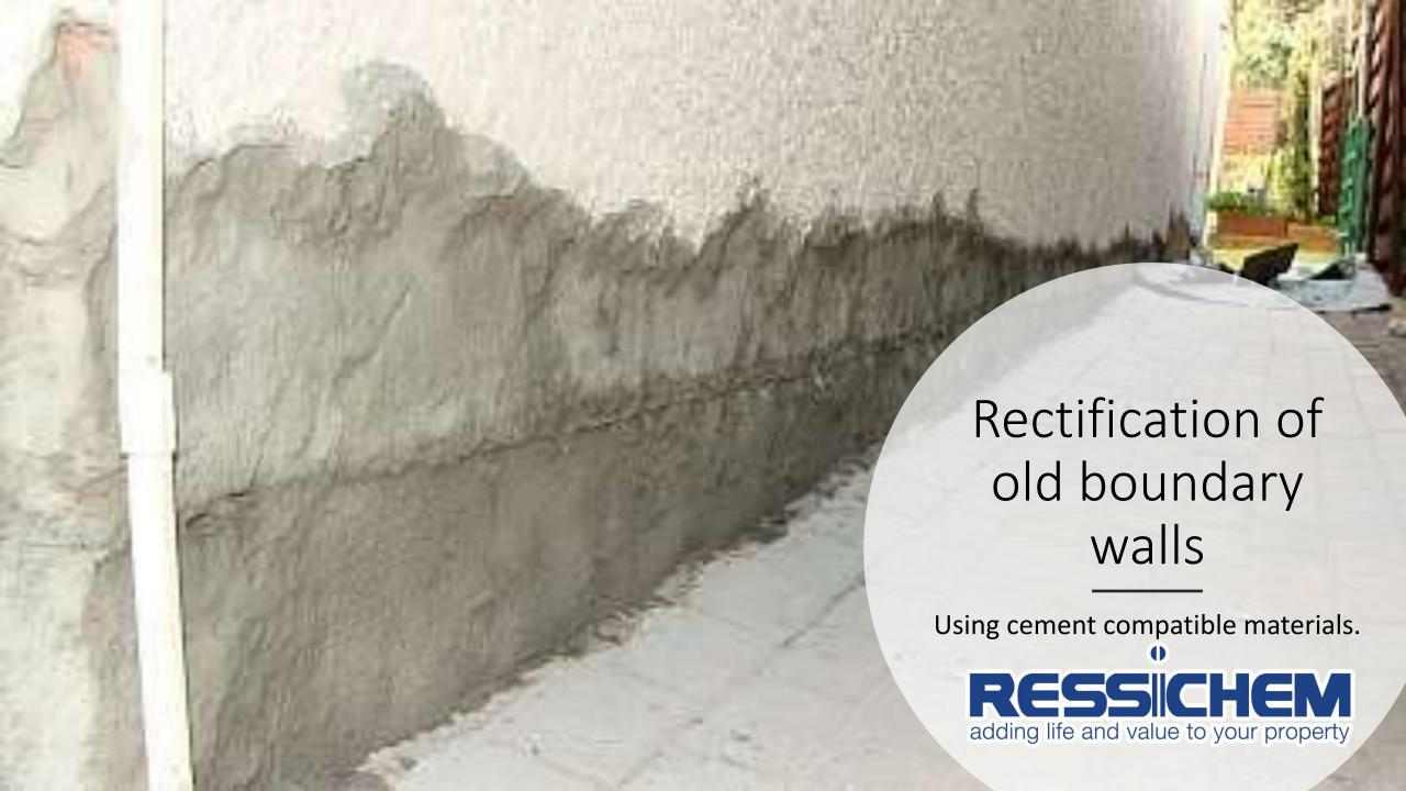
Removal existing plaster from entire surface exposing the brick / block works.
