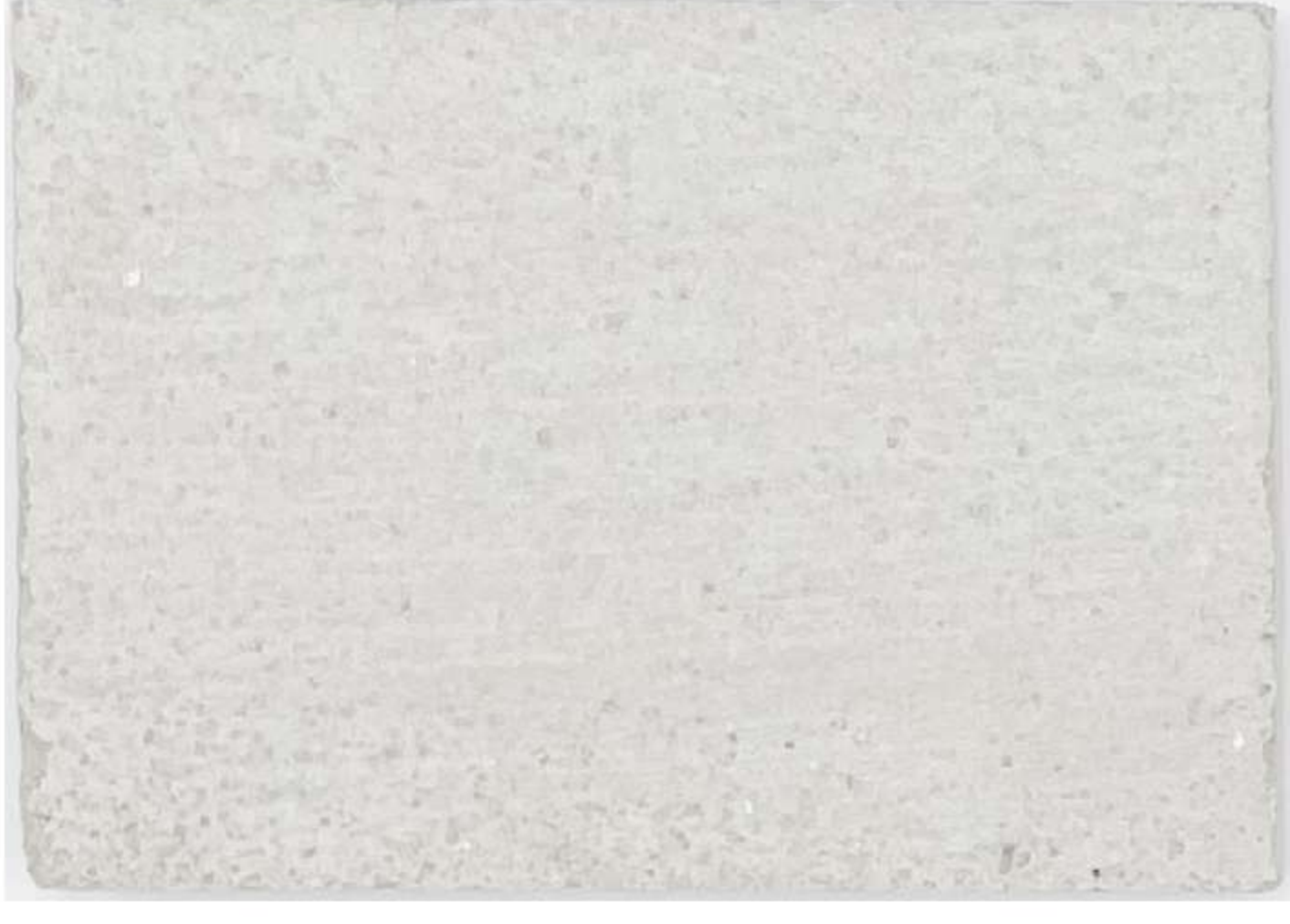
RPR 110-7000 W (Fair Face Concrete)
