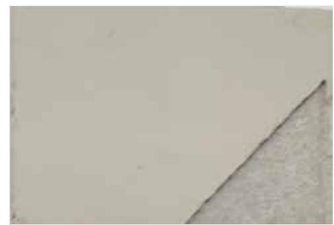
RDR 7000 W (Fair Face Concrete)
