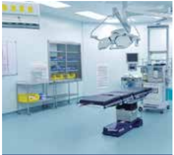
Hospitals Operation Theaters & Corridors
