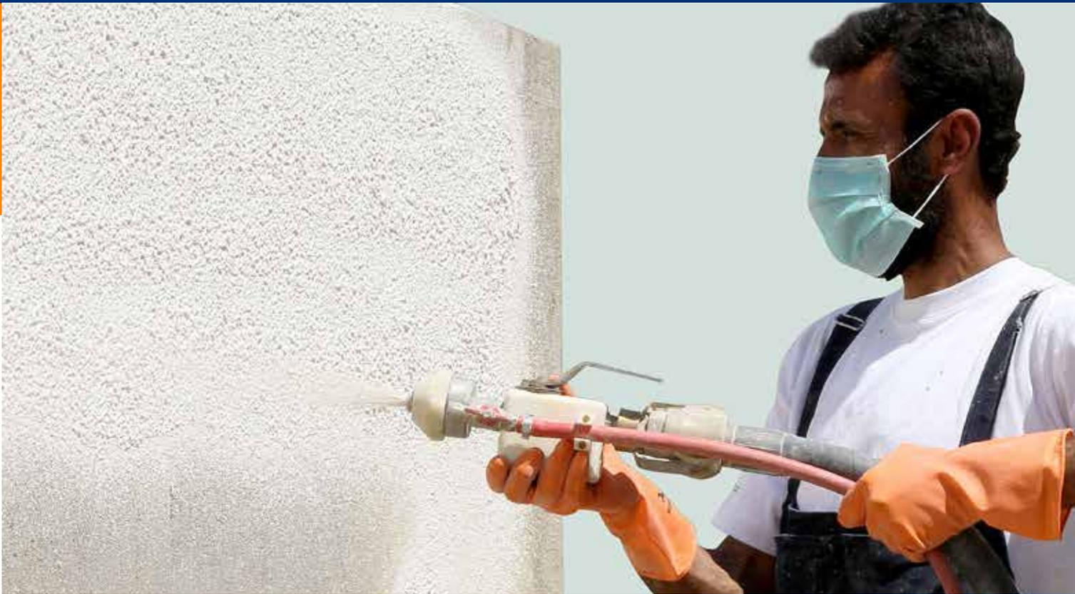
Ressichem Dry Mix mortars / Premix Plasters are factory manufactured dry mortars conforming to specific mix proportions of ingredients e.g., Binders, Aggregates, fillers, pigments, chemical additives, etc.
